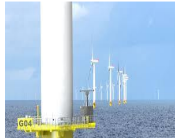
Radar system on transition piece
