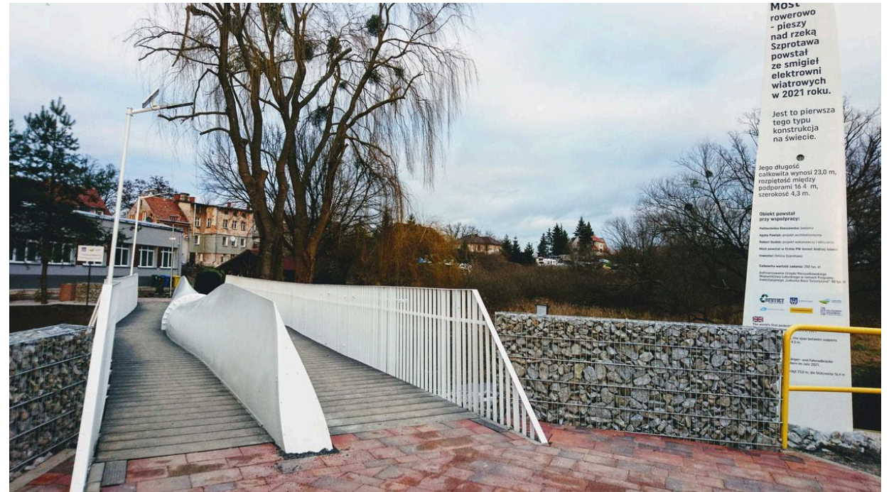
[2] Amnet's worlds first turbine blade bridge, Szprotawa, Poland 2021
