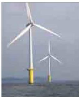
1 North Hoyle Offshore Wind Farm Project
